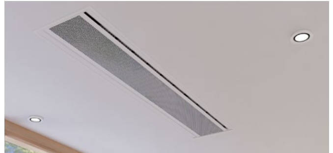
Figure 9. WISE Pacific with Plasterboard frame, PACIFIC T-FPB
